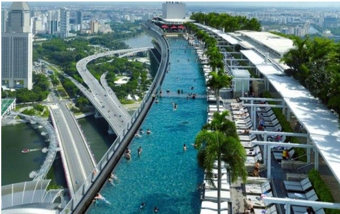
Singapura – Piscina suspensa no hotel Marina Bay Sands
