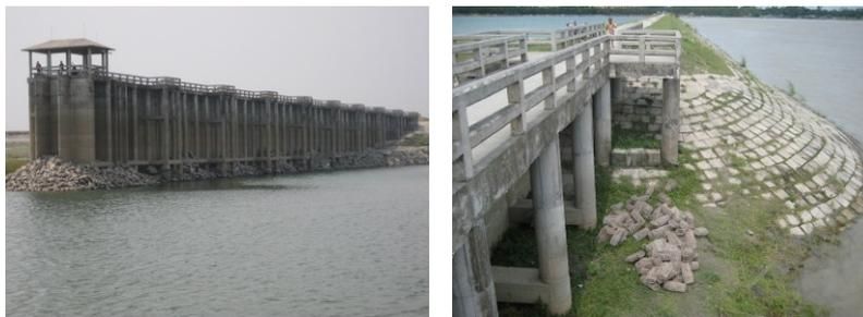
**Fig. 2.** RCC part and earthen shank of the Betil spur
